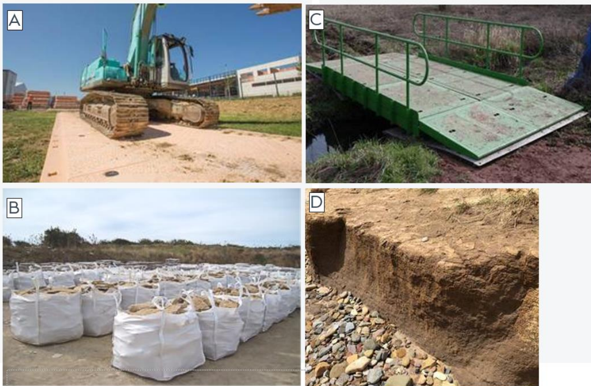
Figure 4.16: Sand bag and access track construction for temporary beach access
